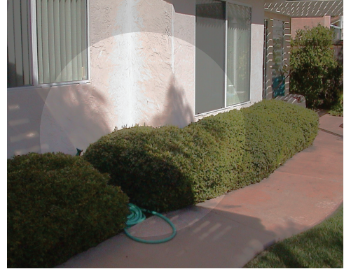
Heavy vegetation against the exterior wall potentially causing moisture intrusion.
