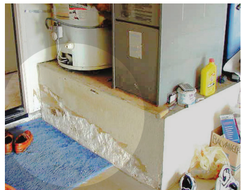
Mold growth and water damage from a leaking water heater on A/C pedestal .
