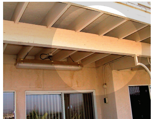
Decking potentially causing moisture intrusion where deck contacts the wall.
