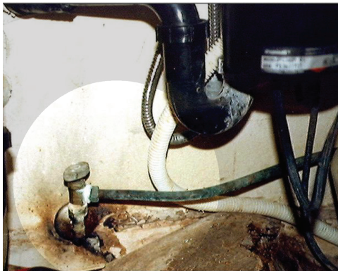
Severe mold growth under a kitchen sink from a leaking supply valve in the wall .
