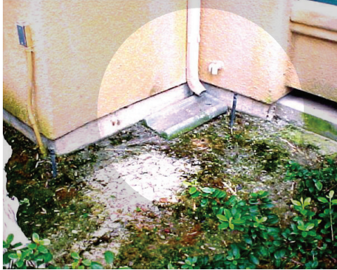
Rain gutter and sprinkler heads located too close to the home. Note algae growth.
