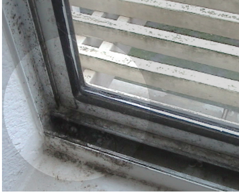
Condensation causing mold growth inside of window tracks and on metal framings.
