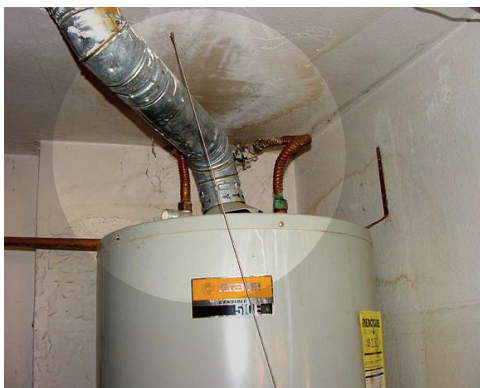
Water damage on garage ceiling from a leaking water supply line .
