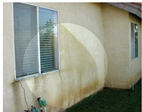
Staining caused by sprinklers spraying the side of the home.
