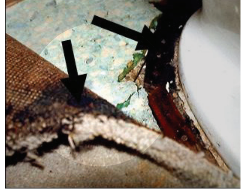
Water damage and mold growth around a leaking wax seal at the base of toilet .
