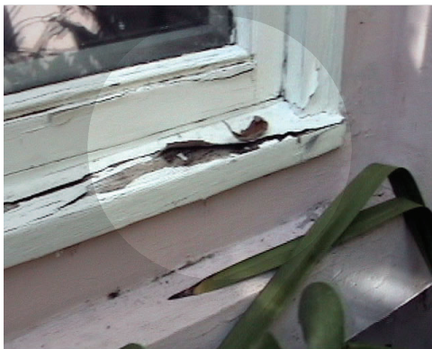
Exterior damage to window sill potentially causing moisture intrusion.
