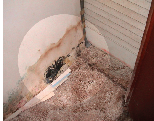
Exterior moisture intrusion causing mold growth and water staining on lower wall.
