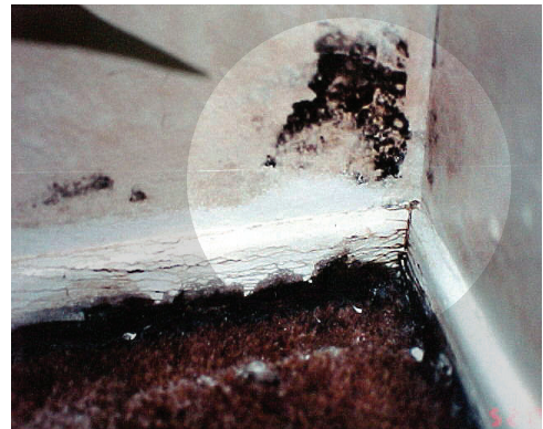
Exterior moisture intrusion causing mold growth on baseboard, wall, and carpeting.
