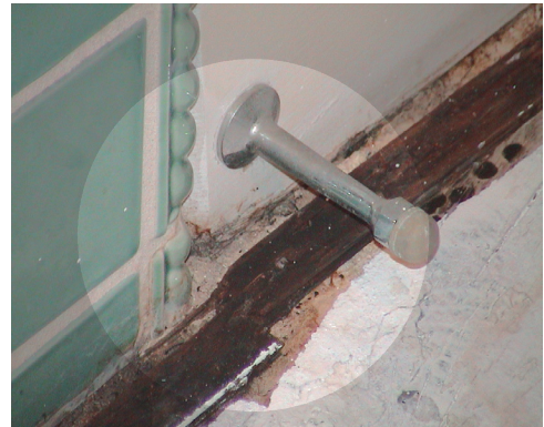
Mold growth and water damage along carpet tack strips in front of a shower .
