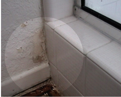
Water damage and mold growth from a leaking shower assembly .
