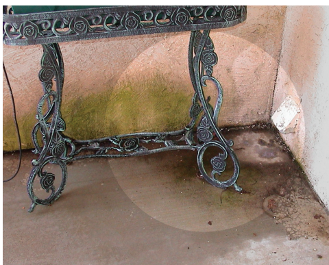
Exterior moisture causing algae growth on stucco wall. Note: concrete patio is covering the lower part of the stucco.
