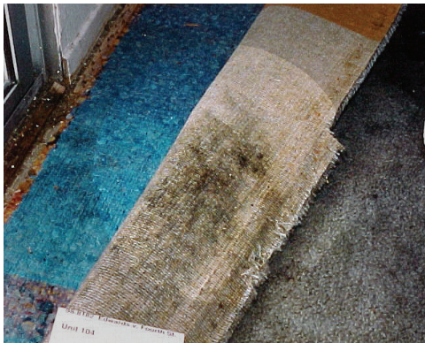
Moisture intrusion under sliding glass door causing mold growth on carpeting.
